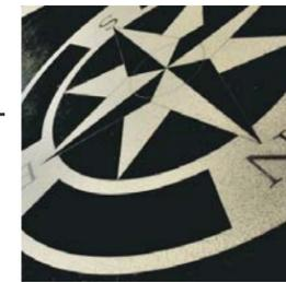
**70%** of the museum quality epoxy terrazzo flooring in the Safety Rest Area is made from recycled glass. Not only does this floor have tremendous long term value related to performance and low maintenance, the usage of recycled glass reduces the amount of glass going to waste, and reduces the need for quarried stone.
