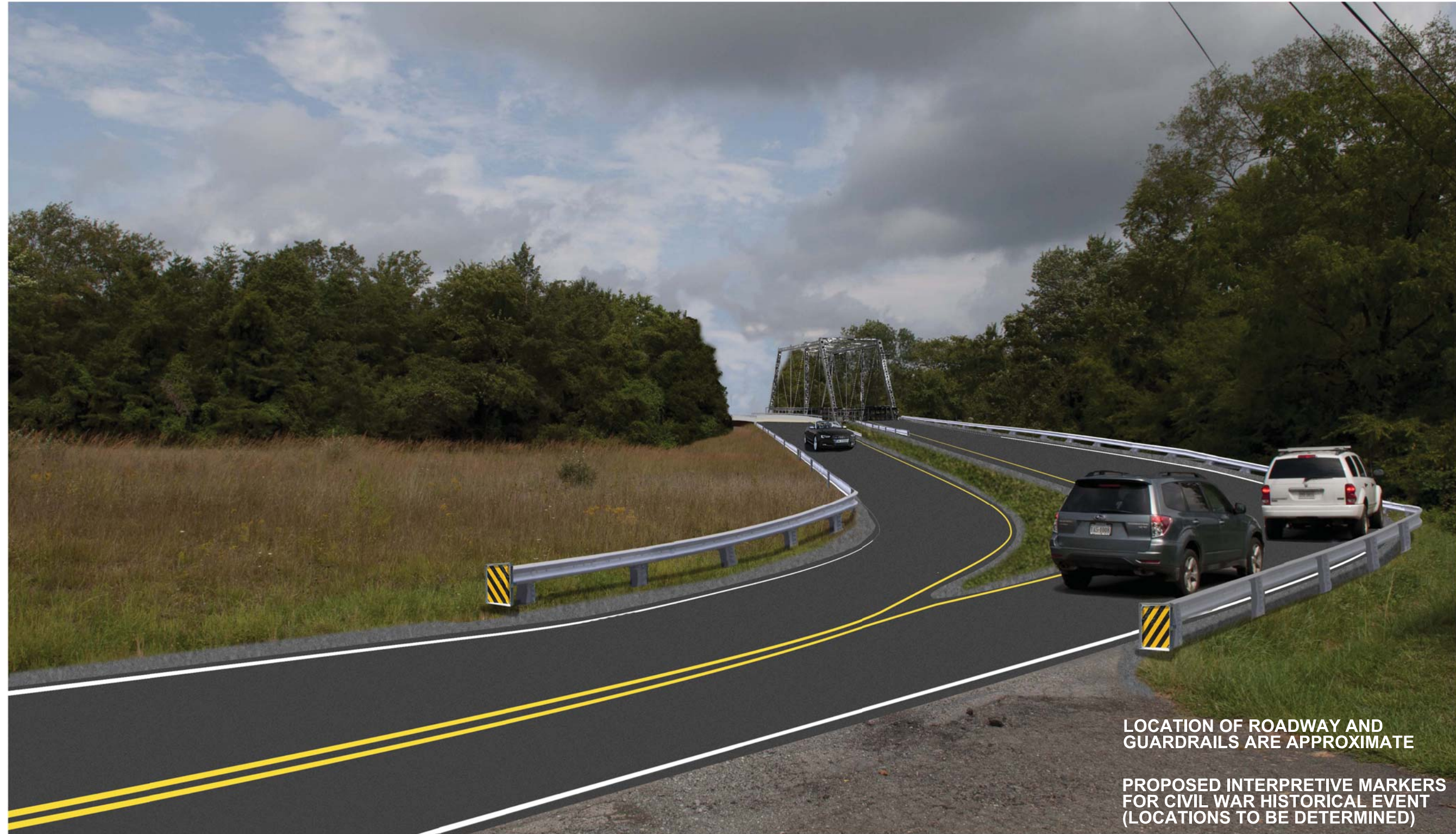
Concept Rendering of Proposed New Steel Beam Bridge (Southbound Lane) & Existing Truss Bridge on New Hammerhead Abutments (Northbound Lane) with Approach Roadway
